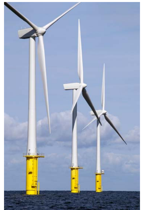
North Hoyle (UK) offshore windmills Photo: Anthony Upton
